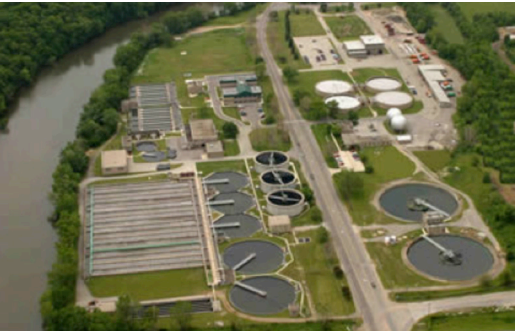
Figure 26 Aerial Image of an Activated Sludge Plant (5 hectares)
