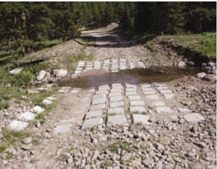
Figure 26 Unvented Concrete Block Hardened Low Water Crossing
